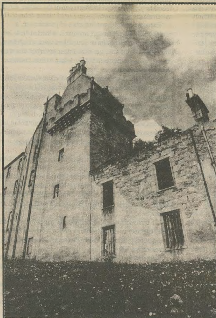
A picture of "Babbettes Tower," Castle Grant, before restoration was begun.
